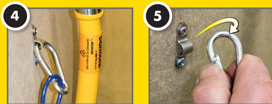
The restrainer wire can now be disconnected to allow free movement of the appliance.
